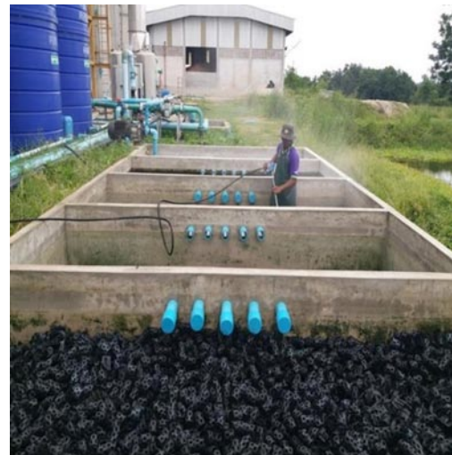
Water recycling system in the wet scrubber system
