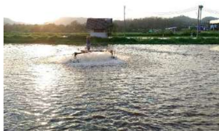
Aerated Lagoon wastewater treatment system
