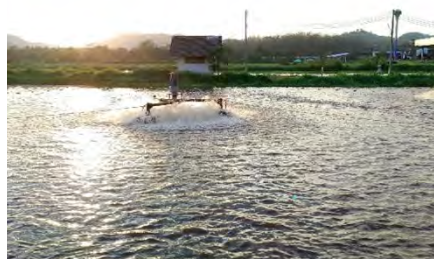
Aerated Lagoon wastewater treatment system
