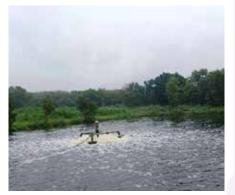
2. Activated Sludge wastewater treatment system is a system that uses aerobic bacteria as the main agents in decomposing organic matter in wastewater in the form of carbon dioxide and water. The treated wastewater flows to a sedimentation tank to separate the sludge from the clear water. The excess sludge will be disposed of further and the clear water in the upper part will be wastewater that can be drained into the environment. This system will be used at factories in the Northeast.
